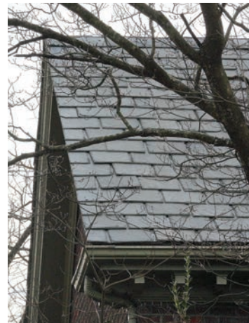
Standard US thickness is 1/4"-3/8", slate is available in thicknesses up to 3/4". 3/8"-1/2" Vermont Blend pictured above.
