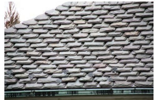
Standard US thickness is 1/4"-3/8", slate is available in thicknesses up to 3/4". 3/8"-1/2" Vermont Blend pictured above.
