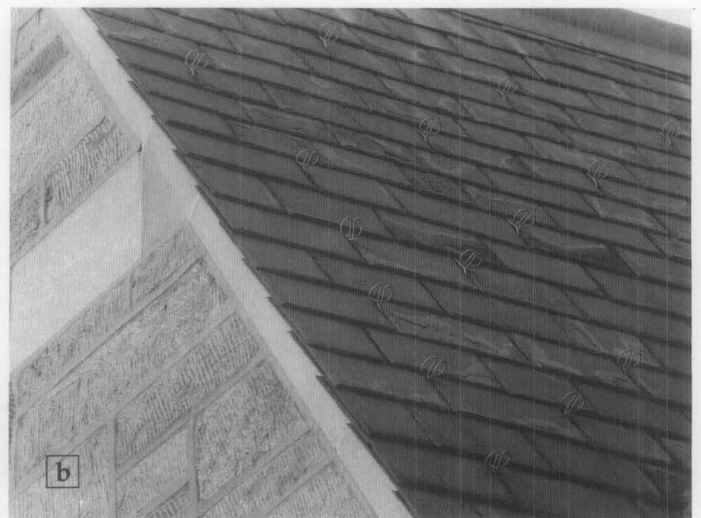
Figure 8. Eave details include snow guards, snow boards, gutter treatments. Snow guards are generally used in areas where ice and snow accumulate to avoid dangerous slides from the roof. In (a) the snow guards are set in two staggered rows above a pole gutter. In (b), the copper wire snow guards are set more frequently up a very steep gable.
