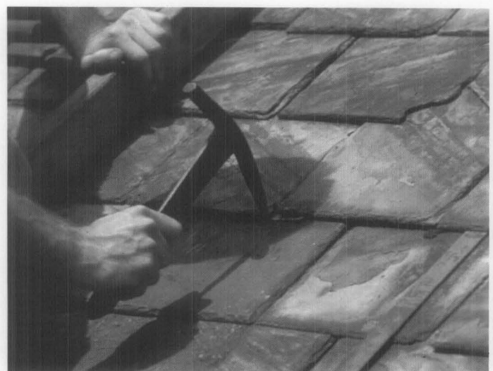
(f) The slate hammer is used to push the bib in place over the nail head.
