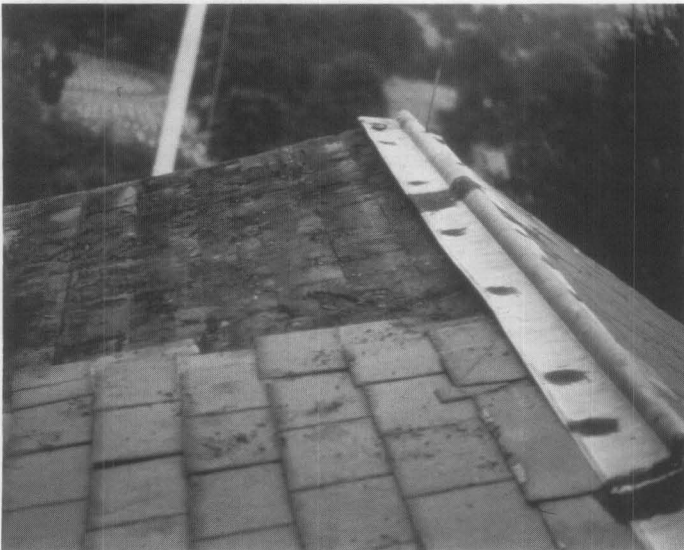
(c) Slate was removed in sections to avoid stress on timber framing.
