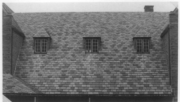
Figure 5. This graduated slate roof is composed of large, thick slates at the eave which are reduced in size and thickness as the slating progresses to the ridge.
