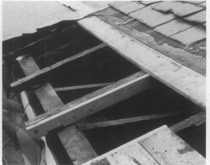
(d) Deteriorated sheathing was replaced and rafter tails were reinforced.
