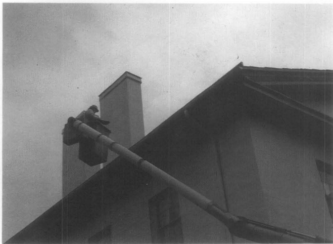
Figure 23. Slate roofs should not be walked on if at all possible. For large projects, lifts can be used to inspect roofs periodically to assess maintenance needs. Photograph courtesy of the National Park Service.
