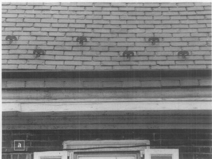
Figure 8. Eave details include snow guards, snow boards, gutter treatments. Snow guards are generally used in areas where ice and snow accumulate to avoid dangerous slides from the roof. In (a) the snow guards are set in two staggered rows above a pole gutter. In (b), the copper wire snow guards are set more frequently up a very steep gable.
