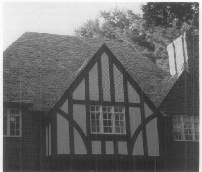
Figure 2. The quaint character of this Tudor style residence is derived, in part, from its textural roof.
