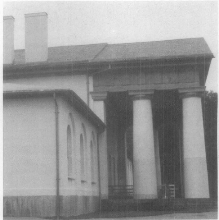
Figure 24. Although slate replacement roofs are expensive, the superiority of materials and craftsmanship will give years of continued service. If amortized over the life of the roof, the replacement cost can be very reasonable. Photograph courtesy of the National Park Service.
