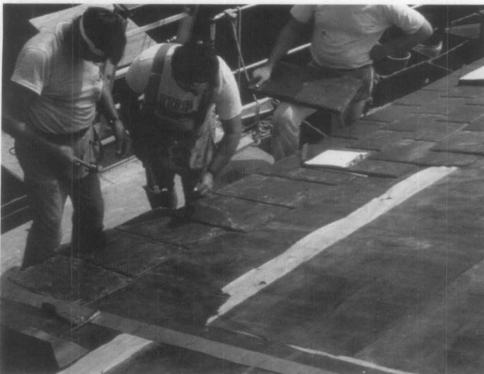
(e) Roofing felt was installed over decking; a rubberized membrane was used selectively at the eaves and under some flashing.
