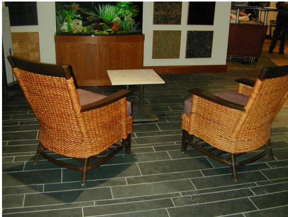
Slate Planking accentuates the stone with the unusual elongated proportions.
