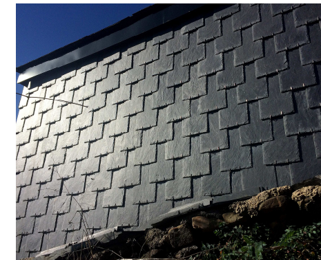
Slate Wall Cladding
