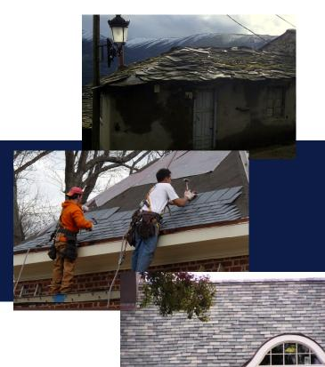
The simple premise behind installing natural slate is a overlapping system. This helps protect the structure and shed water, the beauty of a slate roof is secondary to its protection.
