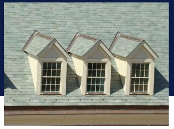
Slate is measured by Length x width in inches. There are over 60 standard sizes in the United States of roofing slate. Slate is then sold in units referred to as *squares*. A square of slate is a 10'x10' area of finished roofing. The smaller the slate the more pieces per square.
